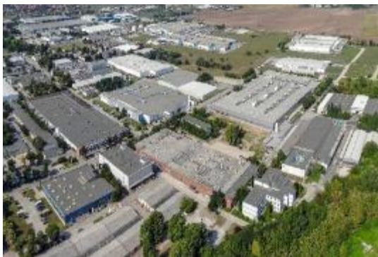
Industrial park services
